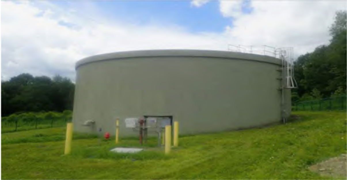
FIGURE 2-4 0.75 MG Prospect Street Water Storage Tank
